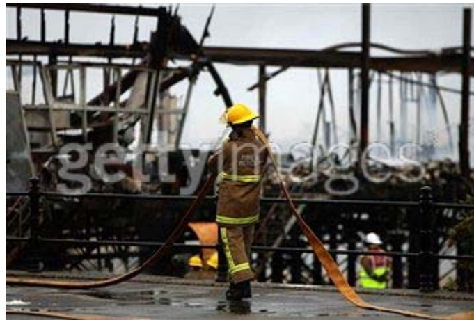
This is the pier after the fire.
